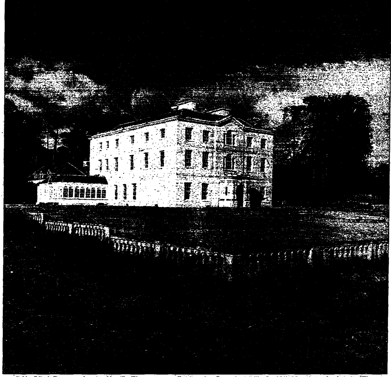
Bridwell Park, Devon, was bought with a £5 million mortgage, suffered a serious fire, and was sold to Lord Ivar Mounbatten for about £1 million
